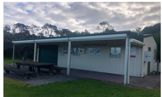
Newly installed blinds at the clubrooms
